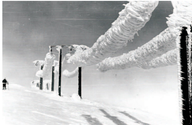
Figure 2.1.5 – Rime on a 22 kV overhead line in Voss, Norway, 18 April 1961 [6]
