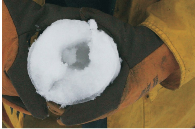
Figure 2.1.3 – Example of Wet snow accretion on a transmission line [3]
