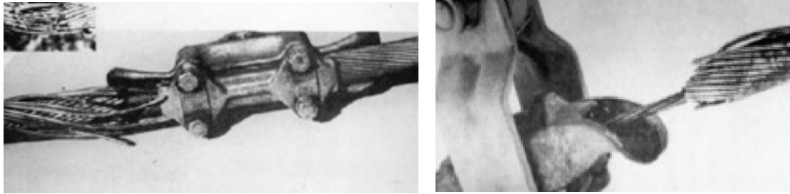
Figure 1.3.2 – Conductors damage at clamp due to fatigue problems [4]
