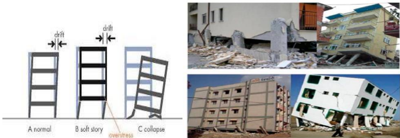
Figure 1-22: Soft-storey mechanisms due to absence at the first floor of the building.
