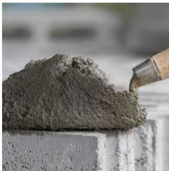
Figure 1-5: Mortar used in brick joints in masonry walls.
