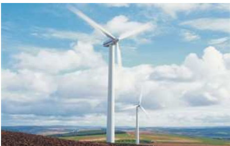
Beenageeha Windfarm, Co Kerry AER III project – 3.96MW Photo courtesy of B9/Renewable Energy Systems
