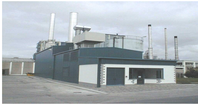
Combined Heat & Power (CHP) Installation at Charleville, Co Cork (AER IV project – 5MW)
