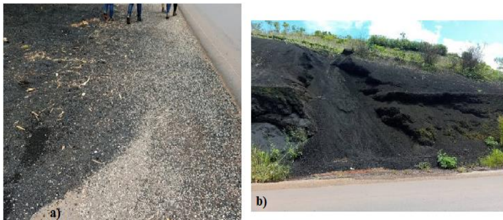
Figure 3.3. Instability manifestations in the black pozzolan deposits
