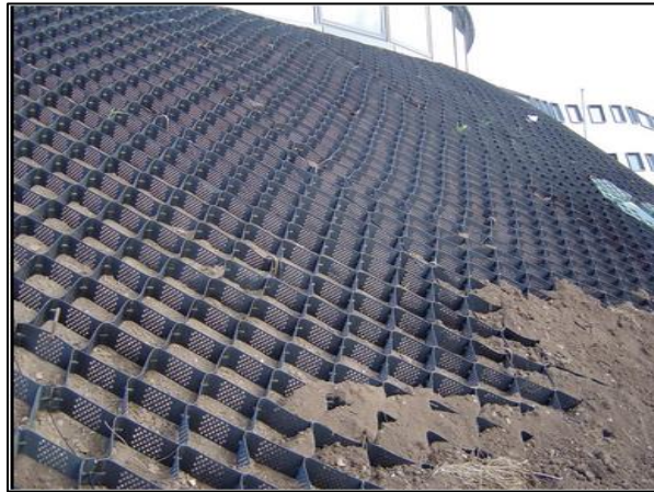
Figure 3.21. Soil confinement system through Geocell (TERRAM Geocell)
