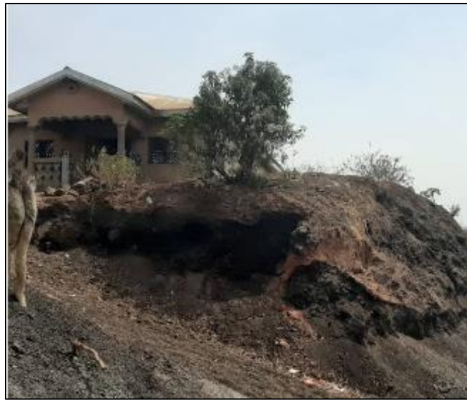
Figure 3.20. House at top of slope at KP 49 of project
