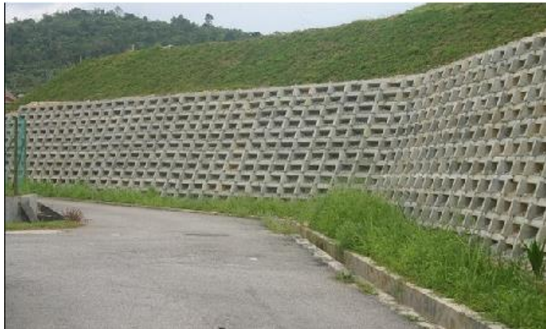
Figure 1.26. Crib wall (Source: CTS BARE)
