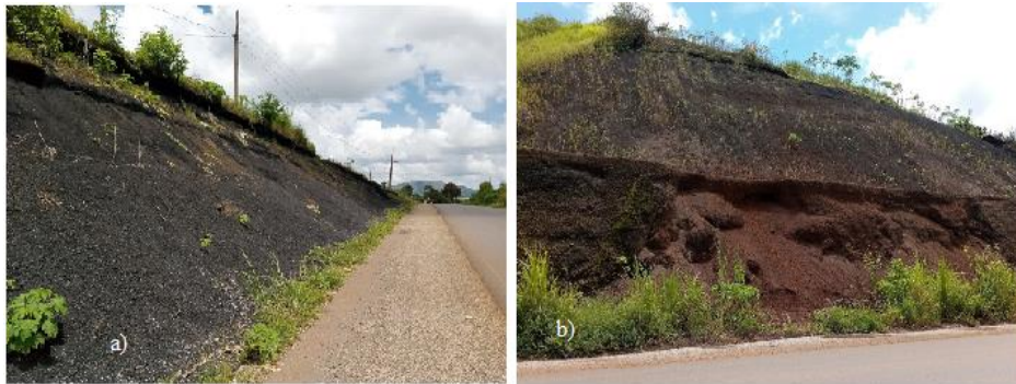
Figure 3.2. Cut slopes in: a) Black pozzolan deposit, b) Red pozzolan deposit
