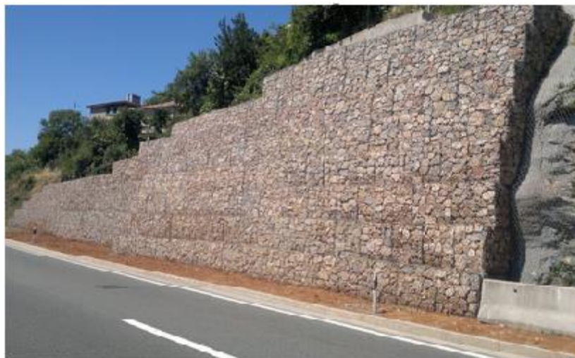
Figure 1.25. cut slope stabilization through gabion walls (Source: Geotech Rijeka)
