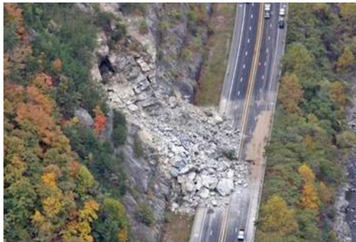
Figure 1.13. Cut slope failure in Bukit Lanjan, Malaysia December 2003 (source: AGU, Advancing earth and space science, 2010)
