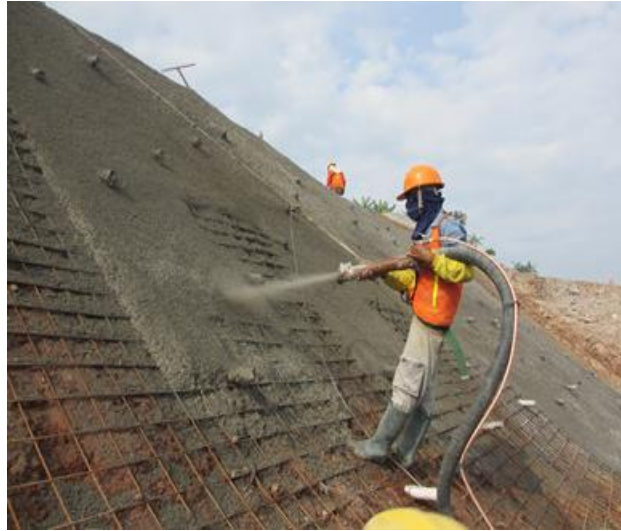
Figure 1.31. Pumping shotcrete
