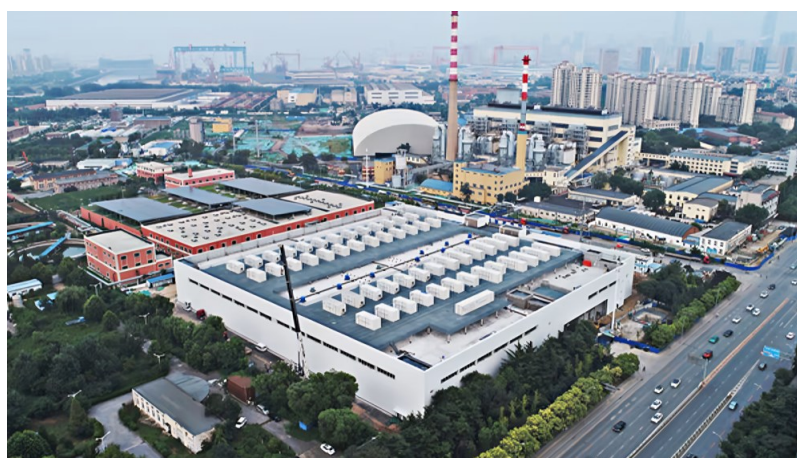
Figure 3.1: Dalian VFB Energy Storage Peak-shaving Power Station. Source: Rinnovabili.it
