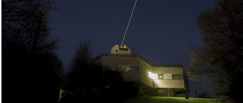
Figure 2.7: Graz SLR station during night operations.
