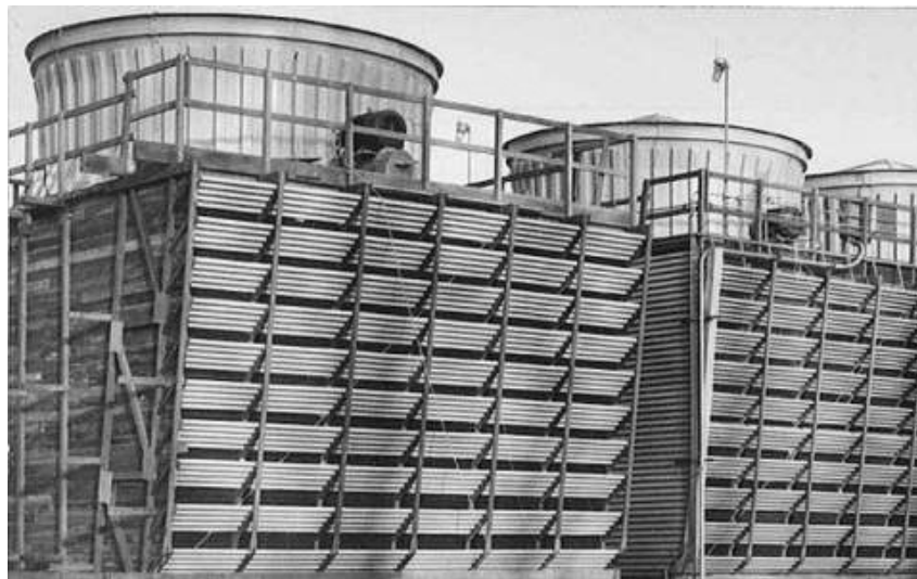
Fig. 2.12: Tower with louvers [6]
