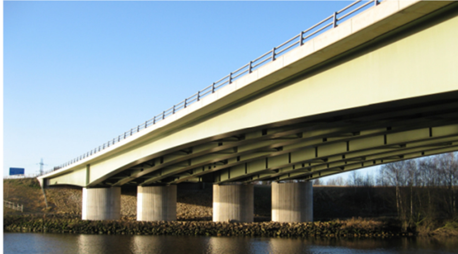
Figure 1.4. Multi-girder composite bridges, Lagentium Viaduct (steelconstruction.info)
