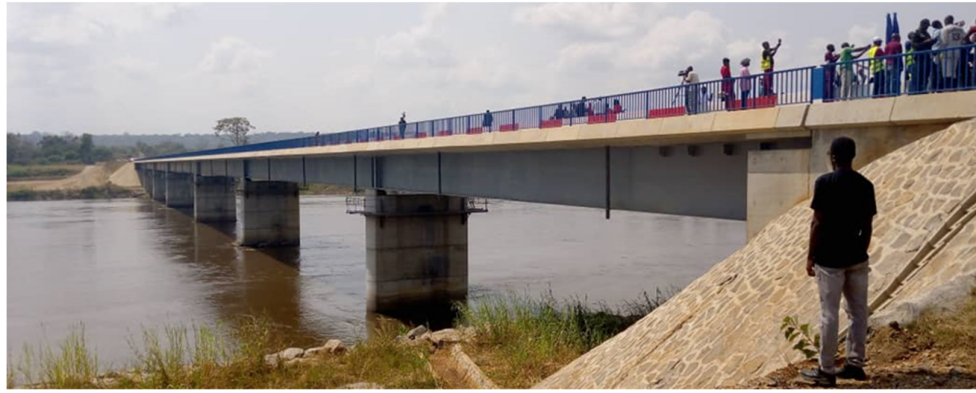
Figure 1.1. Batchenga – Ntui bridge (direct-info.net)
