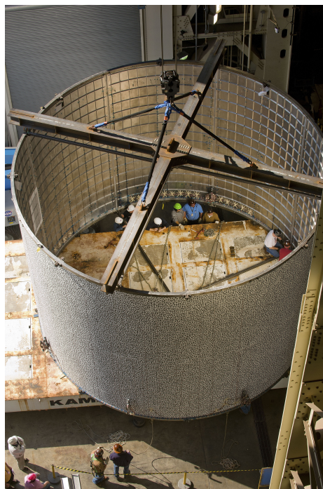
Figure 5.5. A fuel tank shell. Image source:[3]
