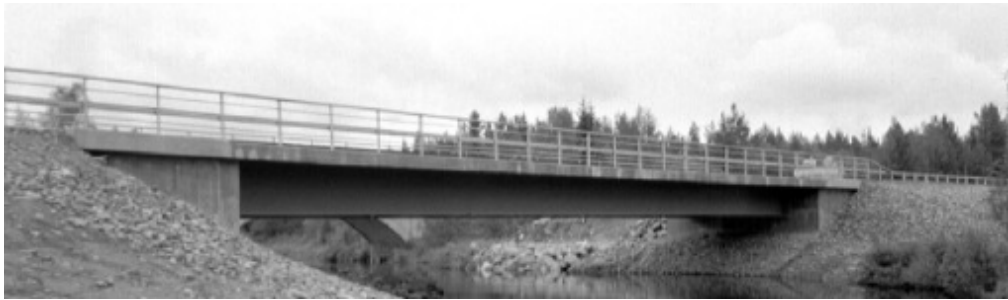
Figura 2-30: Fjällån Bridge (Economic and durable design of composite bridges with integral abutments, 2010)
