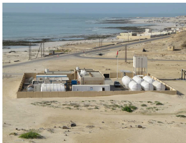
Figure 1.19: The freshwater production plant at Al Khaluf, including MOD plant [29]
