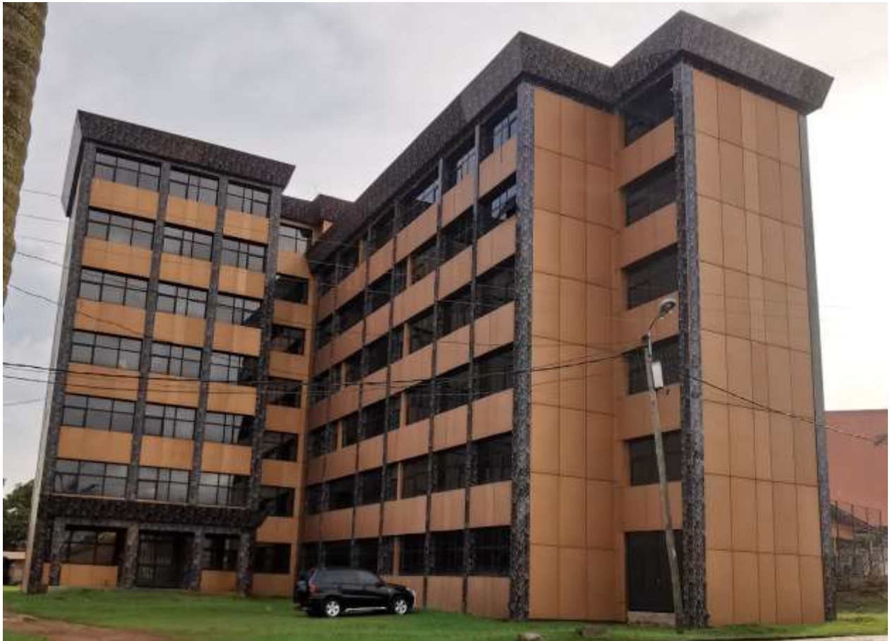
Figure 3.1. Administrative building in the NASPW Yaounde
