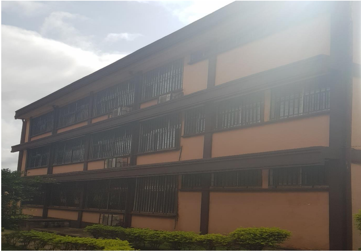
Figure A 1. NASPW Block H building back view
