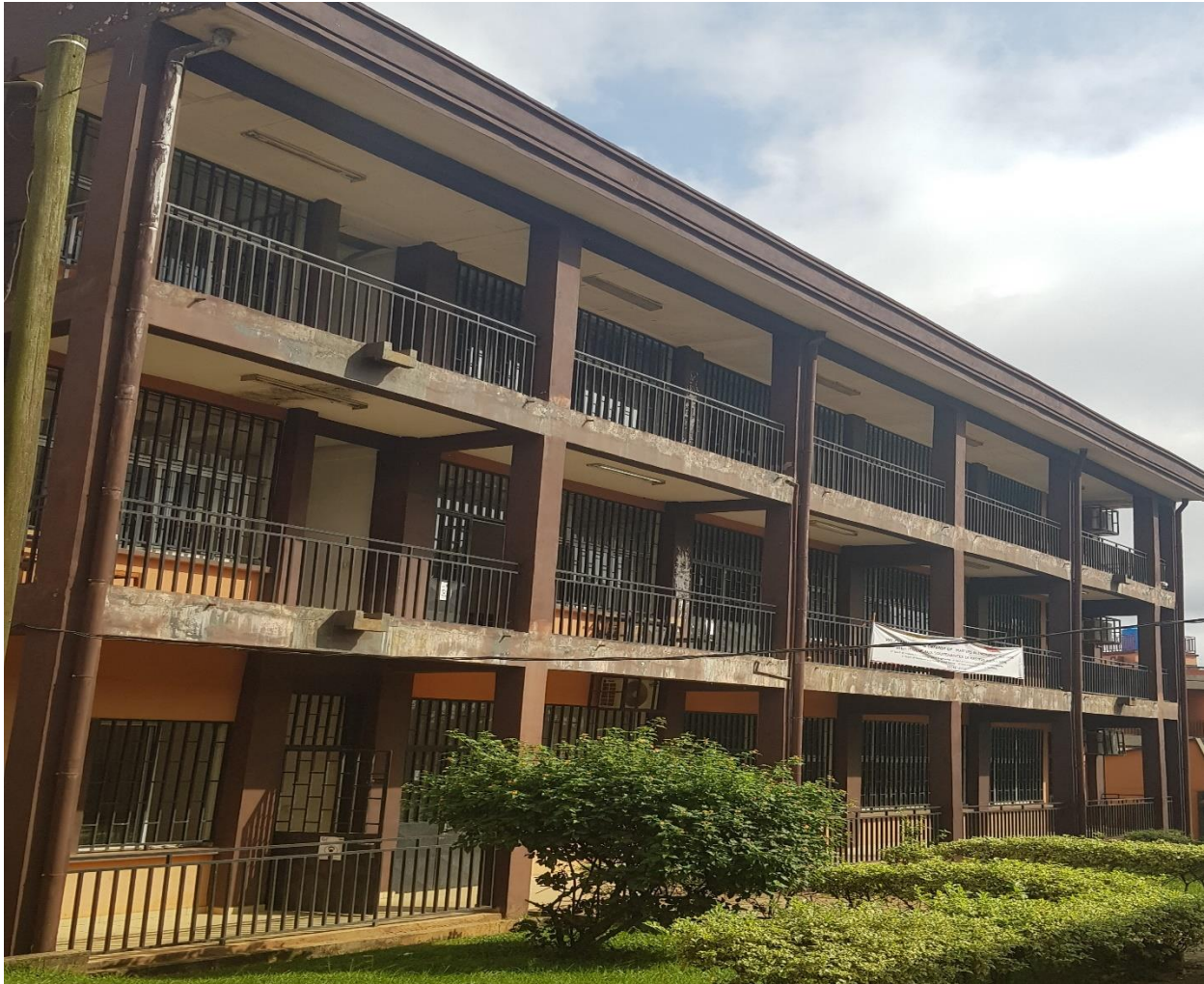
Figure 3. 1. NASPW Block H building front view
