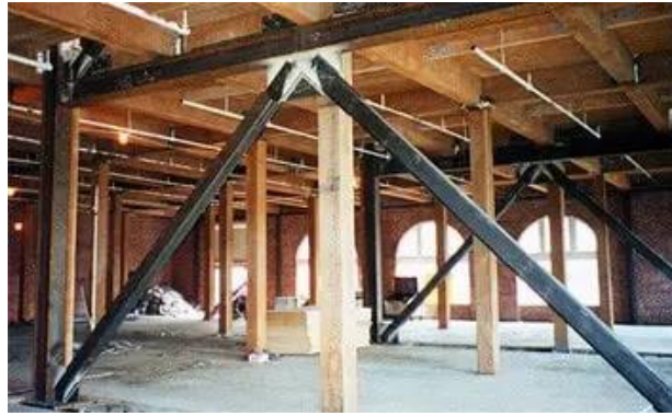
Figure 1.10. Retrofitting by steel bracing support (Bhushan, 2022)
