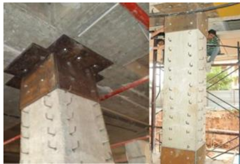
Figure 1.16. Shows a practical example of a steel jacking column. (Chandrakar et al., 2017)
