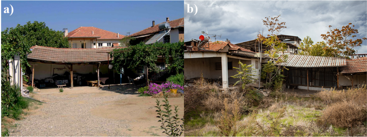
Figure 6.1. Comparison photos of land subsidence in the Sarıgöl district for same location (for photo locations, see Figure 2.3-6). a) Photographed by Demirtaş (2008). b) Photographed by Yüksel (2024).
