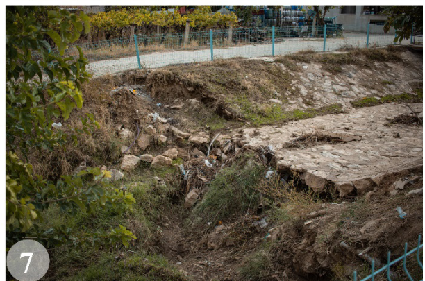
Figure 2.4. Visible earth fissure photos from Sarigöl district (photos by Can Yüksel, 2023)
