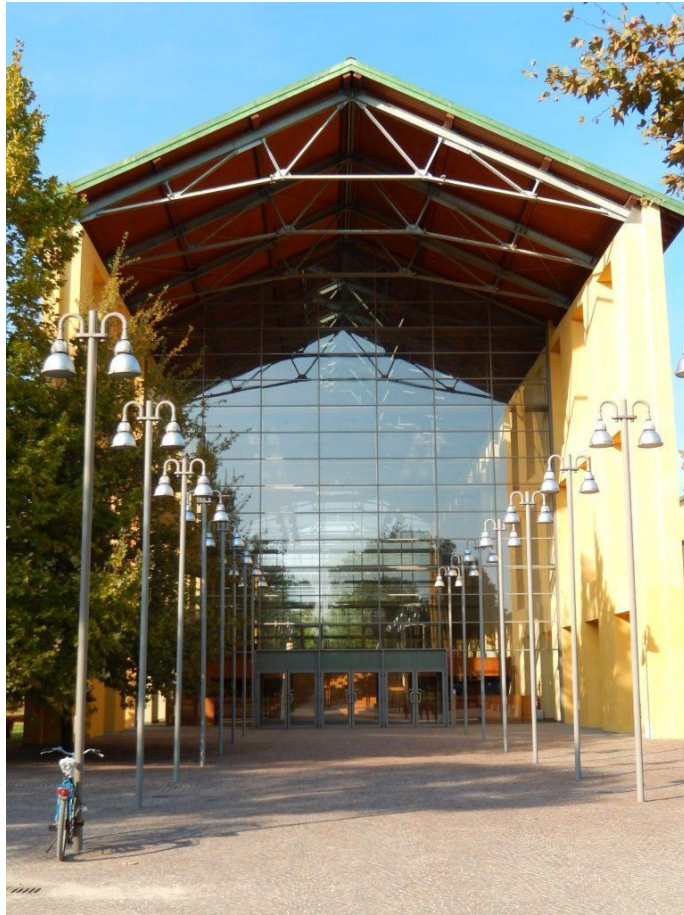
Fig. 10 – Prospetto principale lato sud, in https://archidiap.com/opera/auditorium-paganini/#gallery-1
