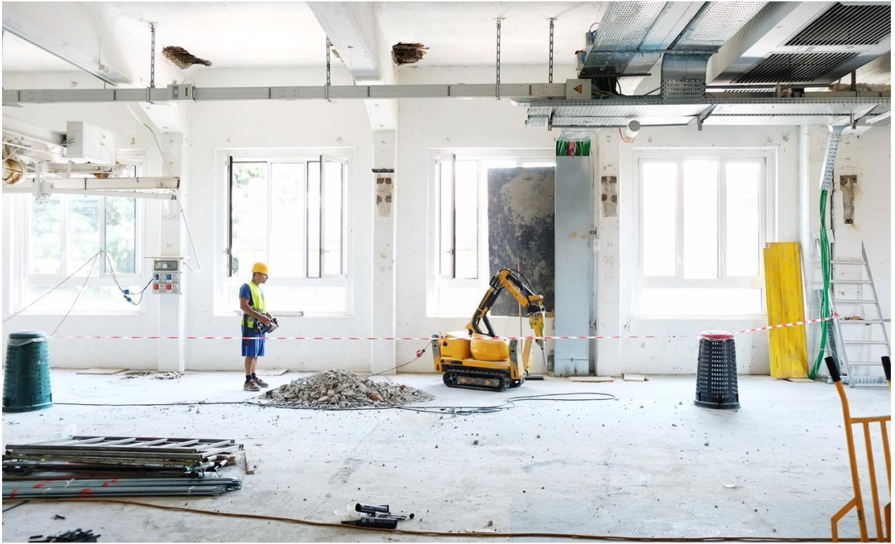
Fig. 7 – Cantiere, in https://base.milano.it/about/
