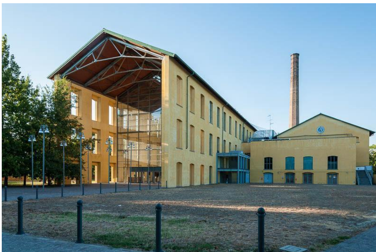
Fig. 12 – Vista esterna del complesso principale, in https://archidiap.com/opera/auditorium-paganini/#gallery-1
