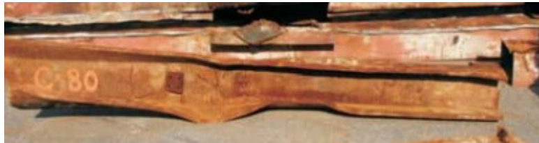
Figura 3.32. Colonna C-80 appartenente al WTC 1 (S.W. Banovic, T. Foecke, and F.W. Gayle (2006), Assessment of Structural Steel from the World Trade Center Towers, Part III: Physical Damage Caused by Impact of Aircraft).
