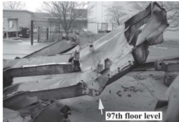
Figura 3.29. Flessione del pannello M-2 in corrispondenza del 97° piano (S.W. Banovic, T. Foecke, and F.W. Gayle (2006), Assessment of Structural Steel from the World Trade Center Towers, Part III: Physical Damage Caused by Impact of Aircraft ).
