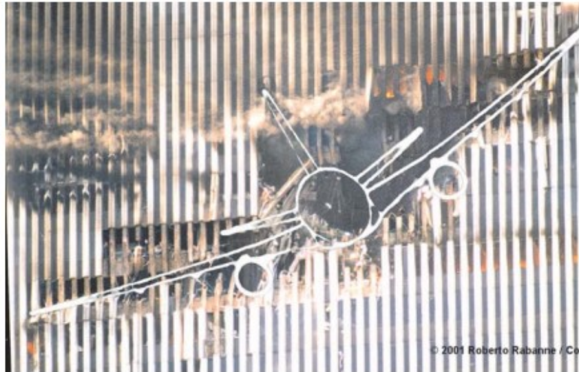
Figura 3.22. Ricostruzione grafica dell'impatto del velivolo sul WTC 1 (S.W. Banovic, T. Foecke, and F.W. Gayle (2006), Assessment of Structural Steel from the World Trade Center Towers, Part II: Analysis of Images for Forensic Information).
