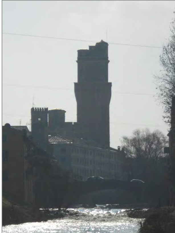
Figure 2-15 Sant'Agostino check dam: downstream view.
