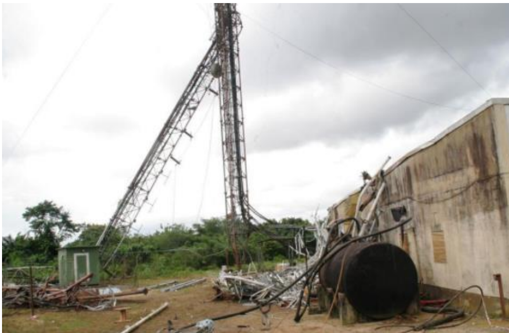
Figure 1.22. Crtv tower collapse in Douala Cameroon 2014. 21
