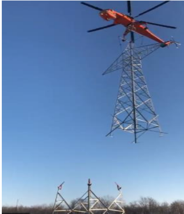
Figure 1.19. Mounting by helicopter. 18
