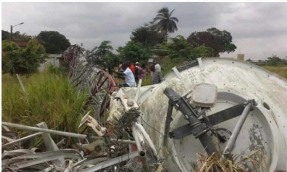
Figure 1.21. Cell tower collapse in the commune of Abobo in Abidjan 2016. 20
