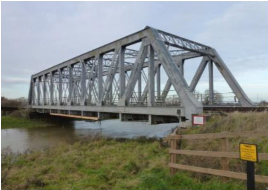
Figure 1.5. Truss bridge (Santosh, 2018)
