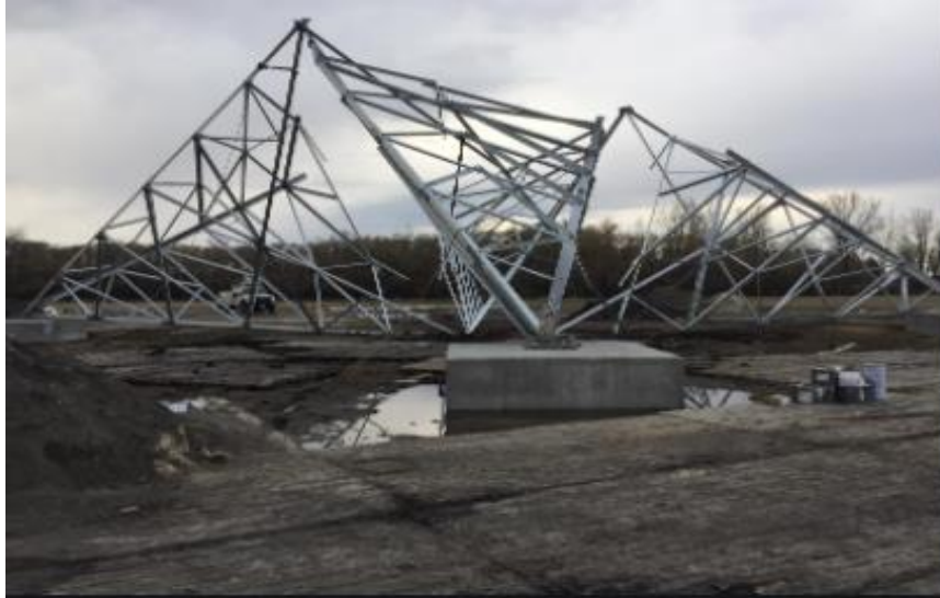
Figure 1.20. Electric tower collapse in Manitoba 2017. 19
