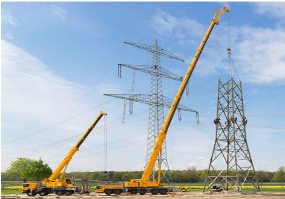
Figure 1.18. Mounting by crane. 17
