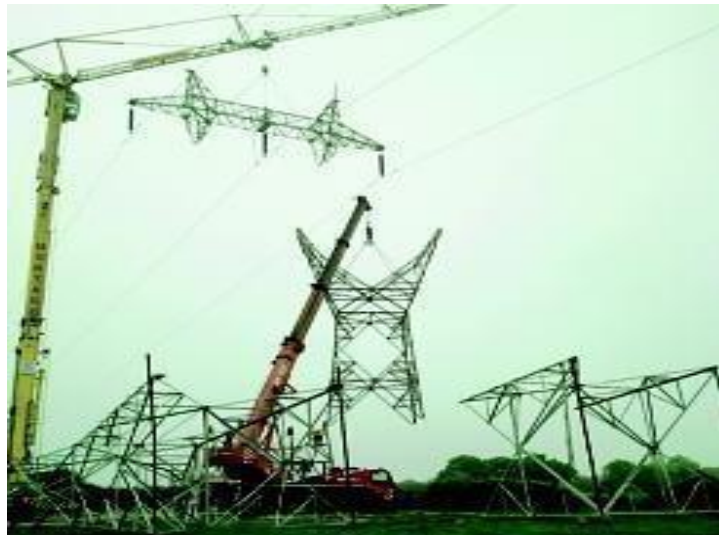
Figure 1.17. Progressive mounting of a tower. 15
