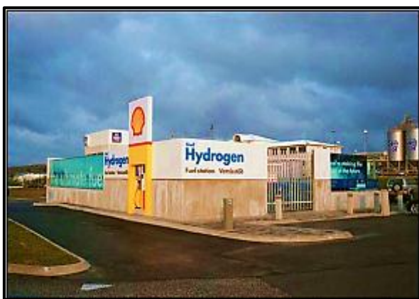
Figura 26. la Fuel Hydrogen Station
