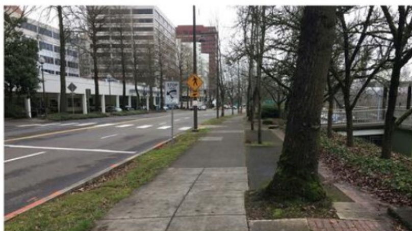
SW Naito Parkway at midblock pedestrian crossing: Existing Conditions
