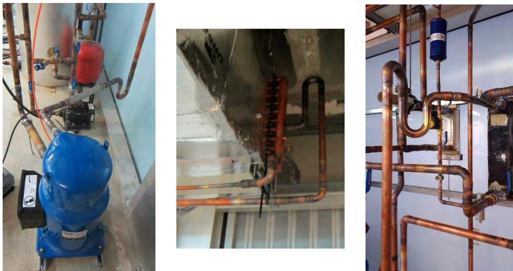
**Figure 31: From the left to the right, details of the flexible sections and elbow downstream the compressor; elbow at the entering of the condenser; syphon after the evaporator.**
