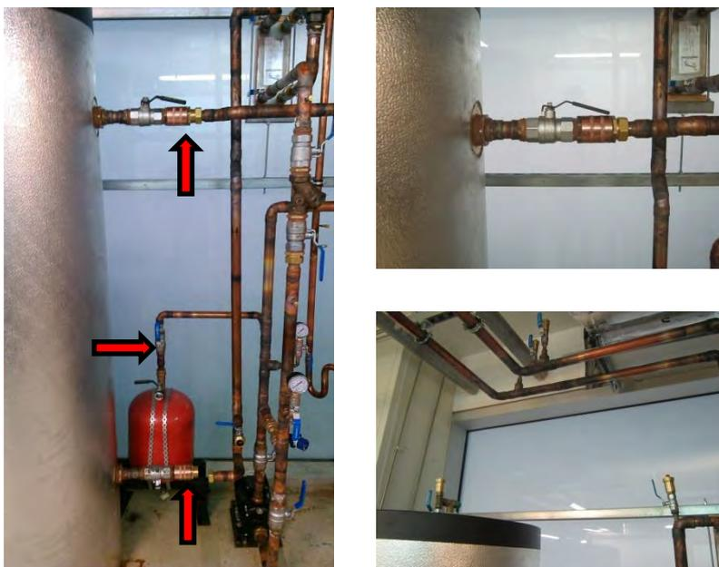
Figure 32: In counter-clockwise from the left, interception valve before the expansion tank and the two anti-electrolysis sleeves, detail of the upper anti-electrolysis sleeve and air purges.
