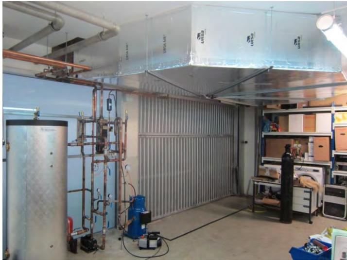
Figure 30: Air conduct above the ceiling and circuit 4 positioning on the left.
