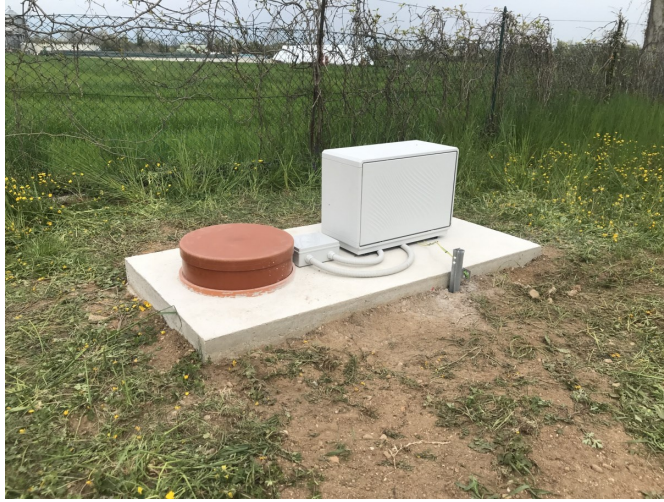
Figure 80: Seismic Station platform built in accordance with SESAME Guidelines
