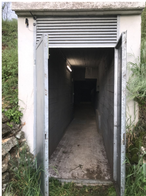
Figure 87: Service tunnel in which the sensor is deployed
