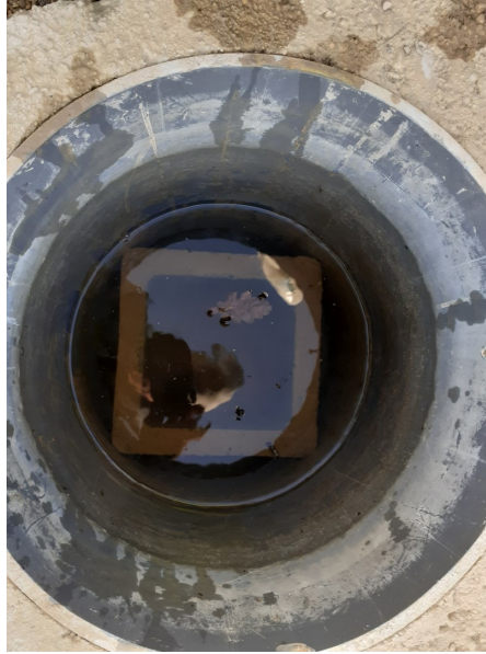
Figure 14: Station 104's seismometer holding barrel - filled with water due to seepage
