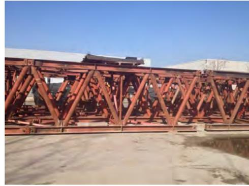
**Figura 399.** *Elemento intermedio  $L = 6,0\text{ m}$  (2/2)*
