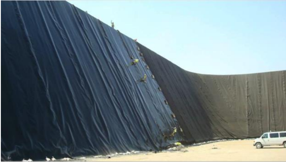
Figure 3.2. Typical landfill geometry with steep slopes.
