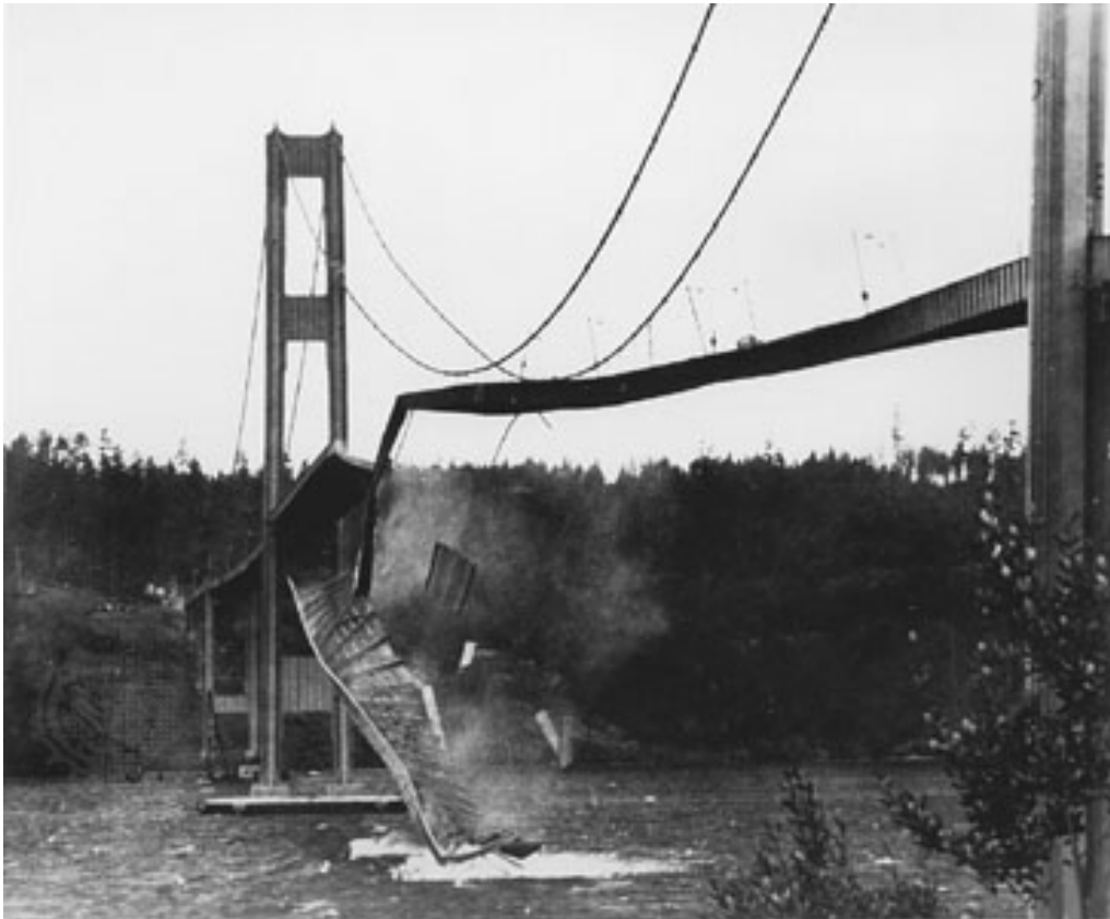
Figure 3.6: Tacoma Narrows Bridge collapsing, November 7, 1940 [26]
