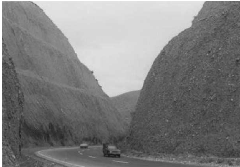
Figure 25. Stable deep trench in the cemented coarse-grained alluvium of Tehran (E. Asghari, D.G. Toll and S.M: Haeri, 2002)
