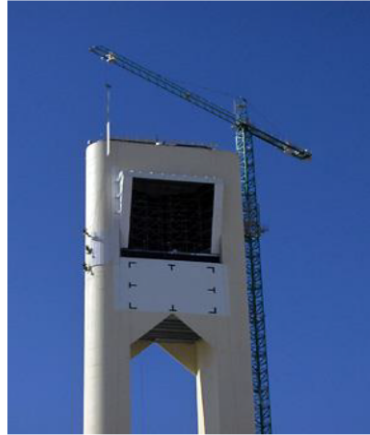
Figure 1.19: Cavity receiver (PS10 plant) [20]
