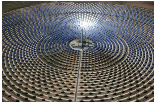
Figure 1.16: Tower in the centre of the heliostat field (Gemastar plant, Spain) [20]
