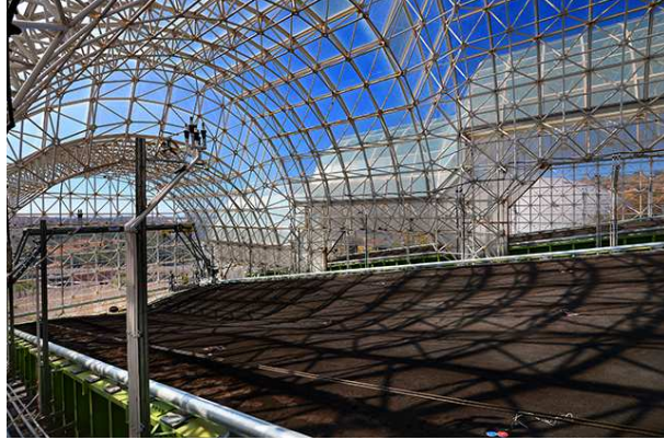
Figure 3.1: One of the three slopes composing LEO facility.
