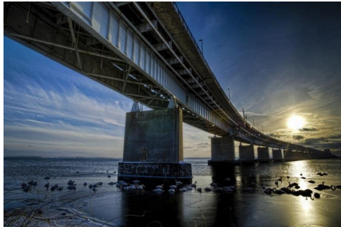
Fig. 2.1: the Storstrøm Bridge
