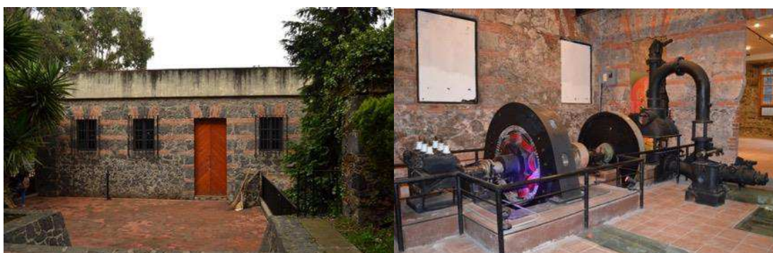
Figure 35. Facade of the building where the dynamo and its interior are preserved.
