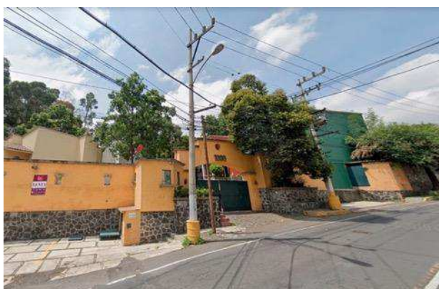
Figure 40. Santa Teresa walls in the Bosque Santa Teresa horizontal condominium.
