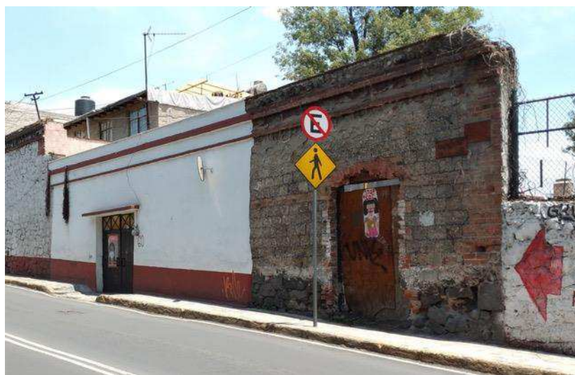
Figure 39. Southern wall of the Santa Teresa factory.
