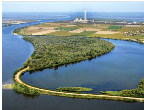
Figure 1.4. Storage basin realized at Volta Vaccari (Porto Tolle, Ro) [16]
