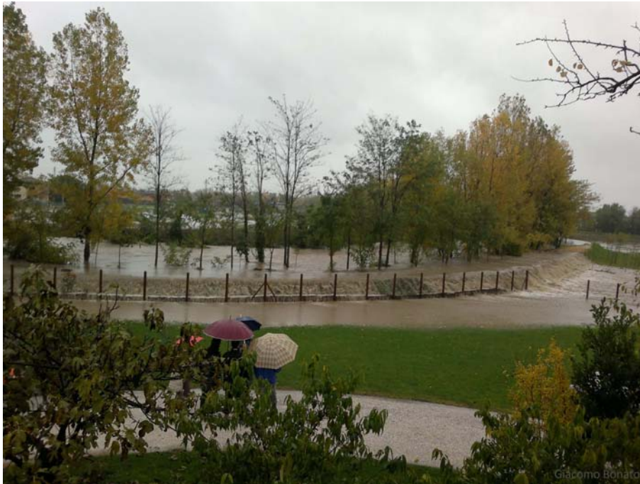
Figure 1.4: Overflow of the embankment at Spineda on November 11, 2012.
