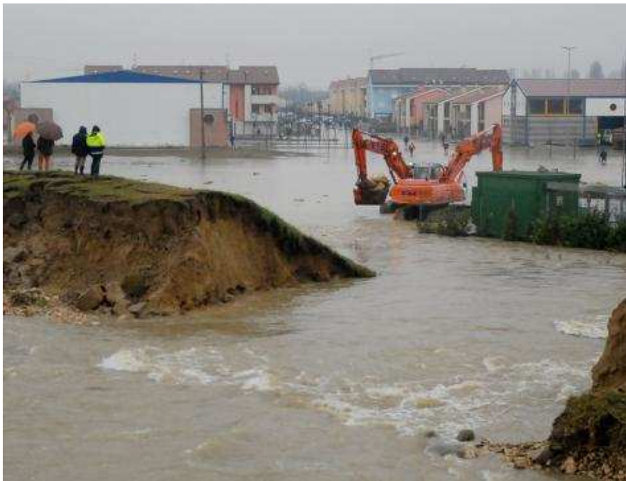
Figure 1.3: Embankment break at Loreggia on January 21, 2009.
