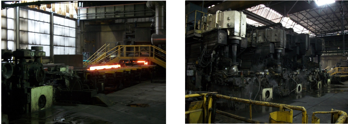
Fig. 6.19b High-lift blooming mill in Valbruna SPA plants
