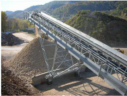
Figure 1.5: Gravel conveyor belt
