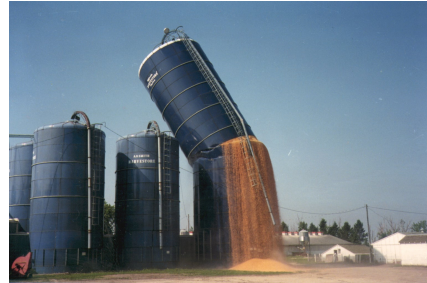
Figure 1.6: Silo failure. This event is linked to the different distribution of pressure in a granular material than in liquids.
