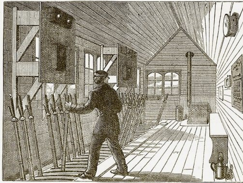
FIG. 48.—Signal-box on the North London Railway
