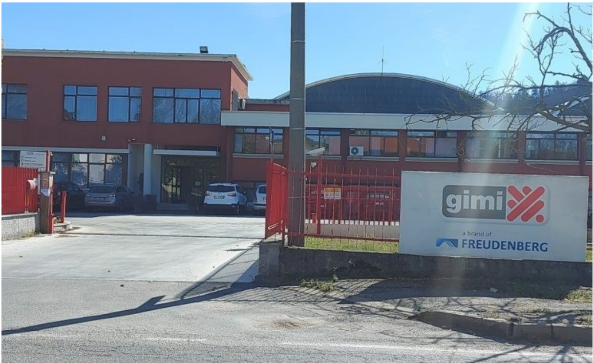
Fig. 27: Photo of the FHP establishment in Monselice
