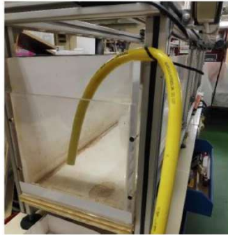
Figure 2.8: Tube connected to the hydraulic system.
