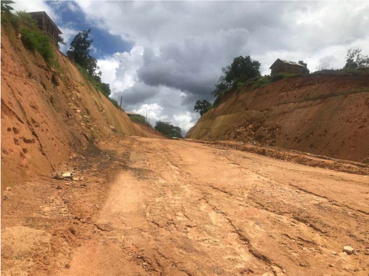
Figure 3.3. Excavated zone showing upwelling by capillarity (Project image)
