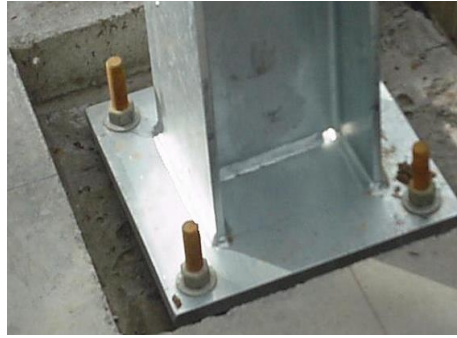
Figure 1.13. Column base plate connection
