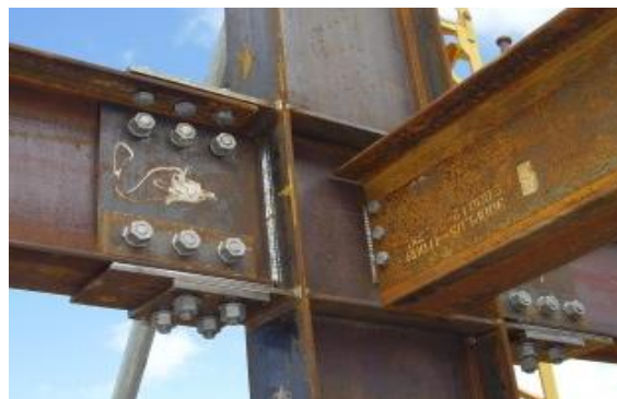
Figure 1.11. Moment connection
