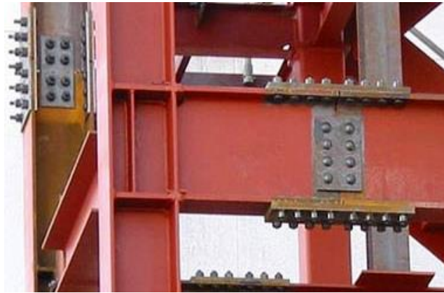
Figure 1.12. Axial connection
