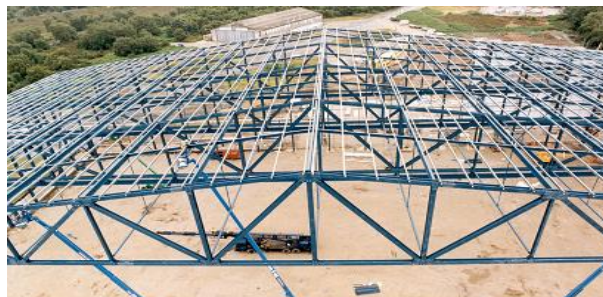
Figure 1.16. Lattice truss structure ( https://www.steelconstruction.info ).
