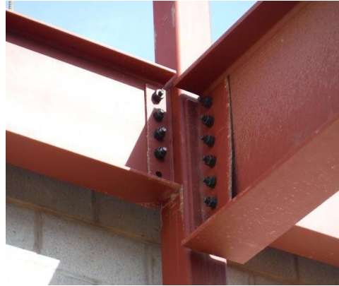
Figure 1.10. Shear connection
