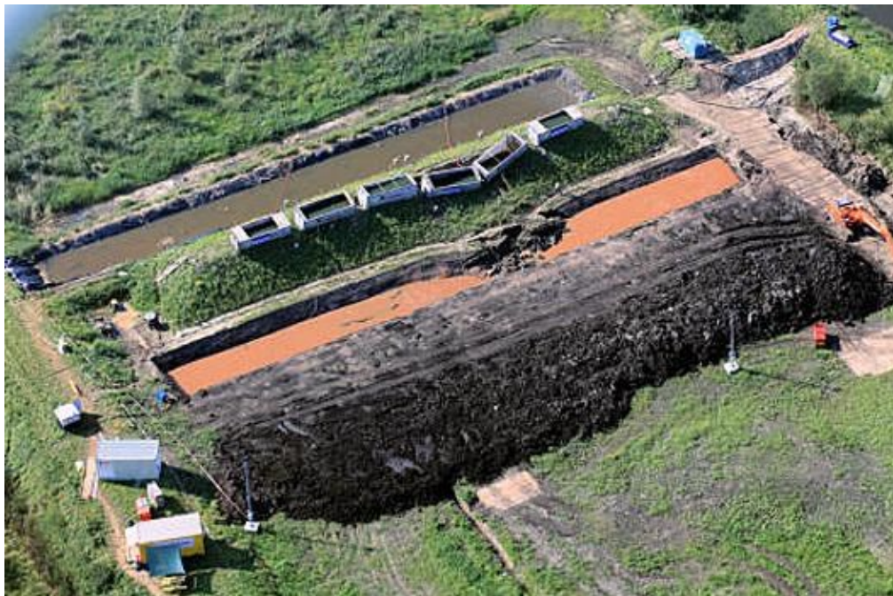
Figure 2. 4. An aerial photograph of the South Dike failure by Boertjens Chose (Zomer, 2012).
