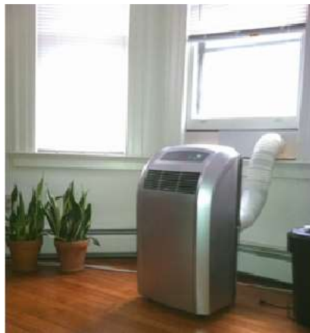
Figure 2.19: Movable single duct unit
