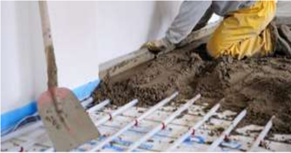
Figure 2.8: (a) High inertia underfloor radiant system, high thickness. (b) Low inertia underfloor radiant system, low thickness – source UPONOR
