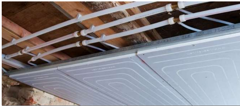
Figure 2.9: Low inertia ceiling radiant system – source Q-RAD
