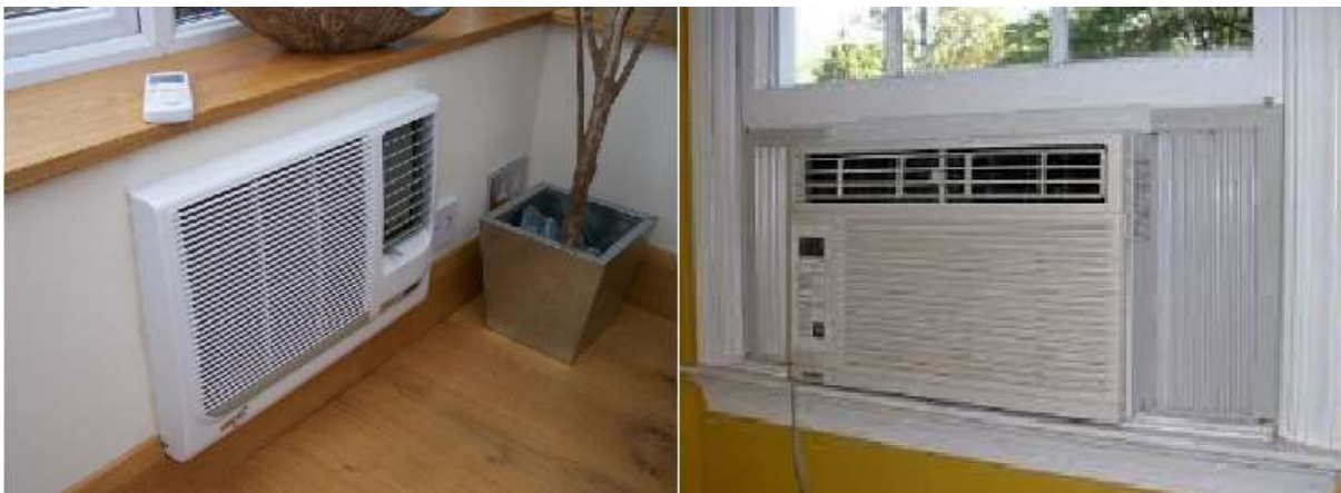
Figure 2.18: Through the wall and window unit's examples
