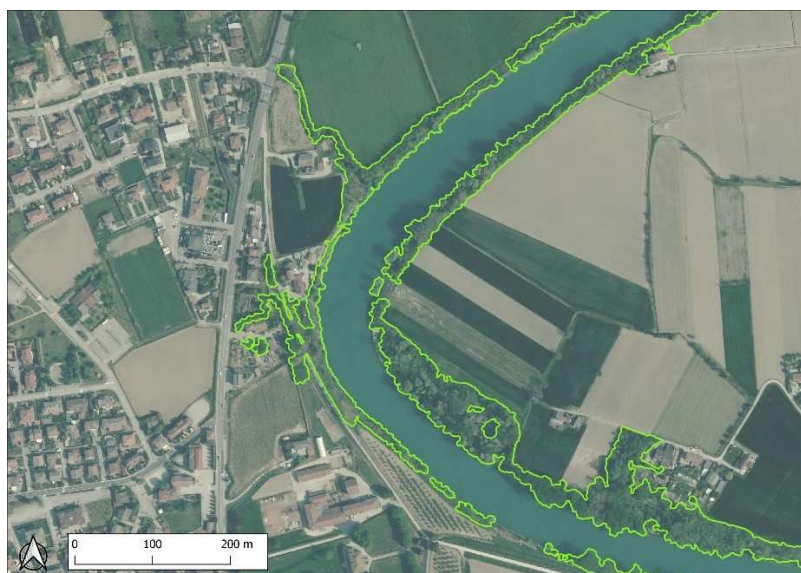
Figure 39. In Vaccarino, the Brenta River crosses cultivated fields on its left, and the dense urban fabric on its right. Consequently, the space for riparian sylvan elements (light green) to expand is significantly reduced.
