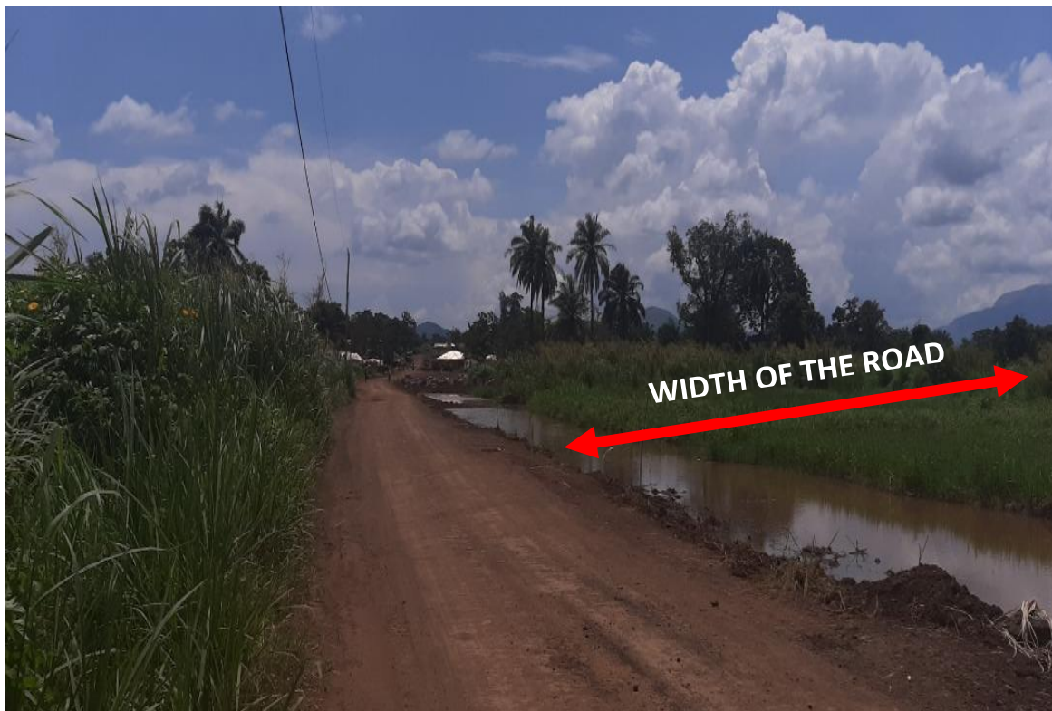
Figure3.5. Initial state of the case study (PK12+900 right)
