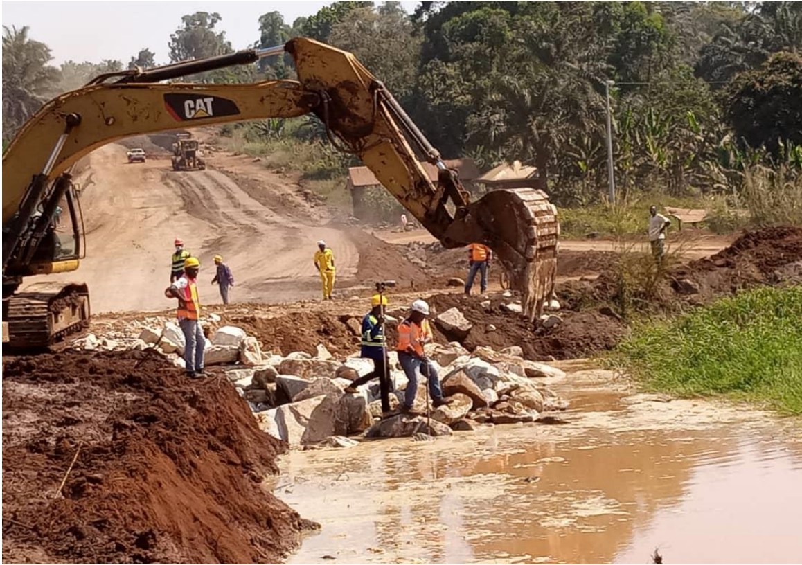
Figure 3.6. Initial state of the case study (PK12+675 right)
