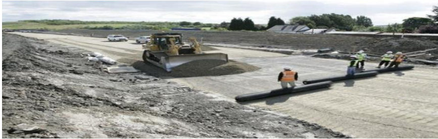
Figure 1.28. Geotextile used in subgrade stabilization. (Source: Geosynthetic international)
