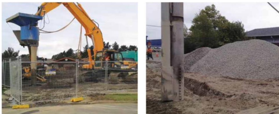
Figure1.20. Stone column realisation
