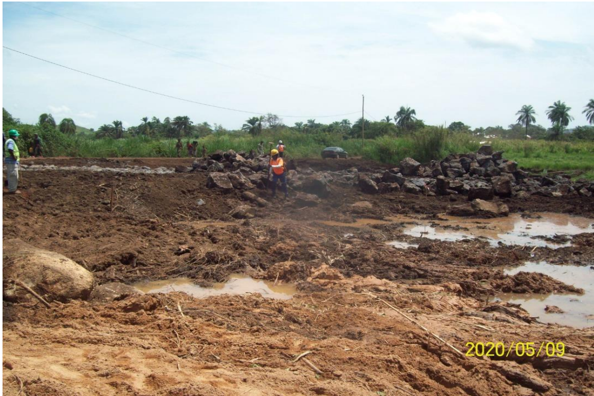
Figure3.4. Initial state of the case study (PK12+900 middle)
