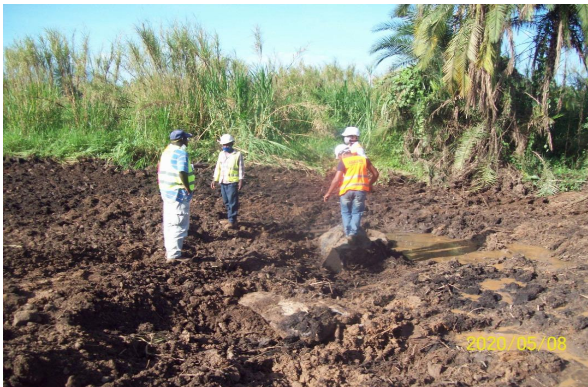
Figure3.3. Initial state of the case study (PK12+650 right)
