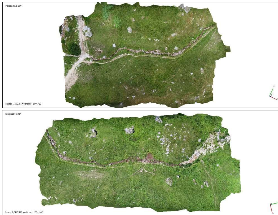
Figure 106: On the upper part the texture of downstream part of "Affluente 3" while on bottom part the upstream part
