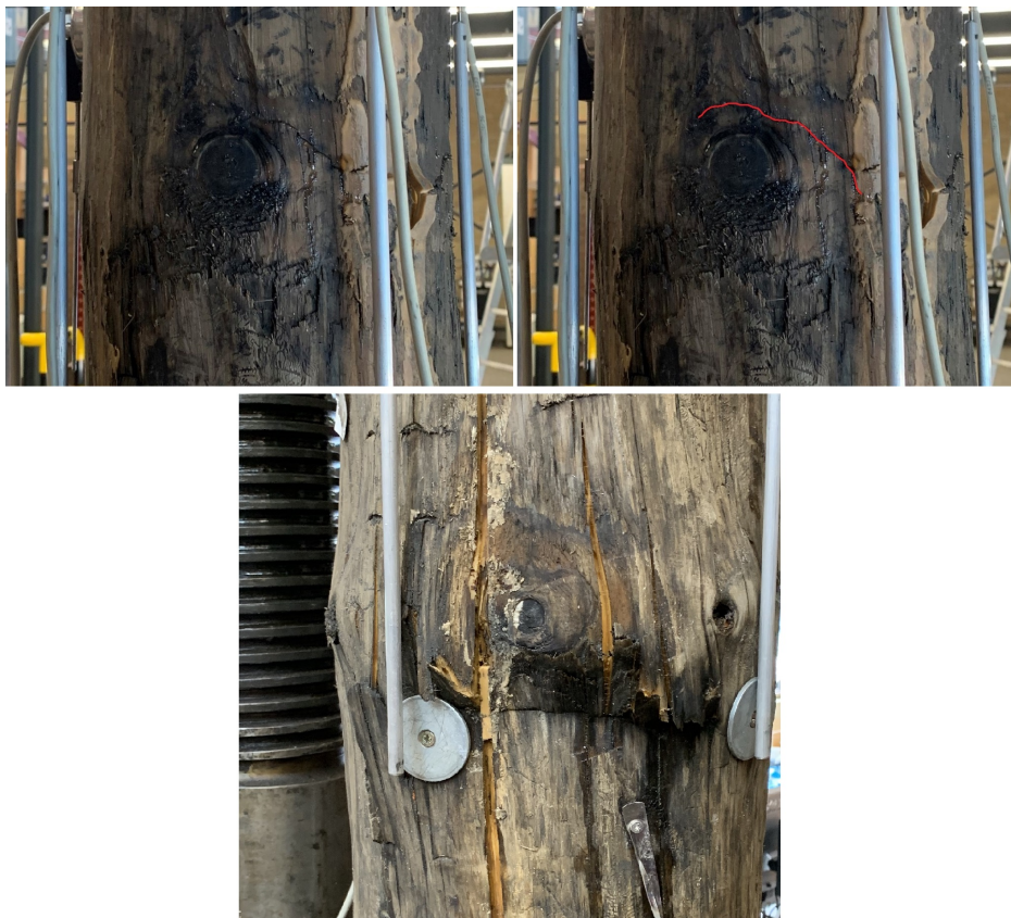
Figure 5.2.4: Failure for localized buckling in correspondence to a whorl.
