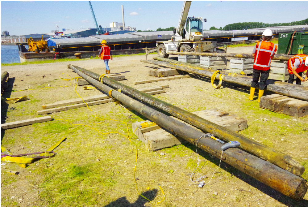
Figure 3.1.4: Piles extracted from the ground in Amsterdam.
