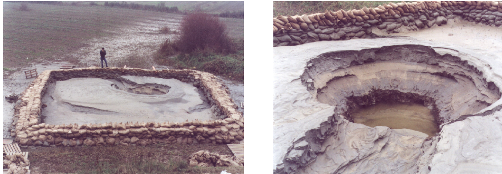
Figure 2.5: Sandbagging around a wide field spring ( fontanazzo ).
