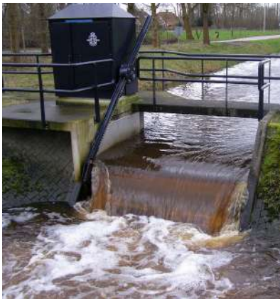
(a) Real weir structure
