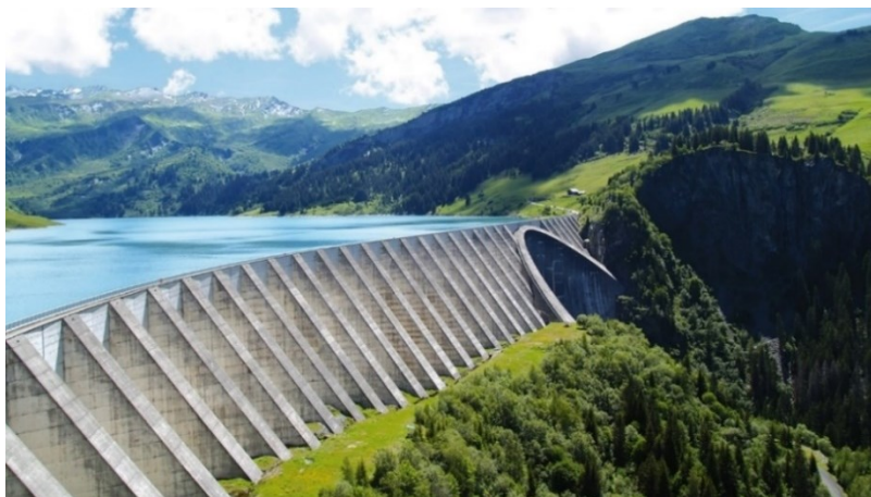
Figure 6.1 Upper reservoir of a PHS scheme
