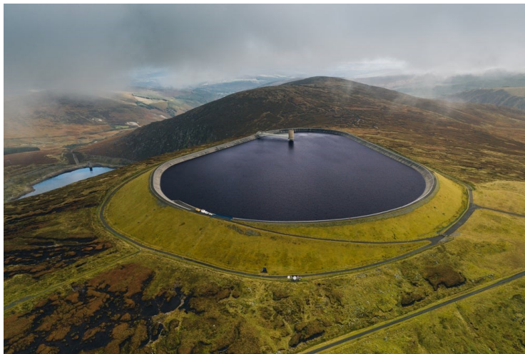
Figure 6.8 A closed loop pumped hydro energy storage station in Ireland's Wicklow Mountain
