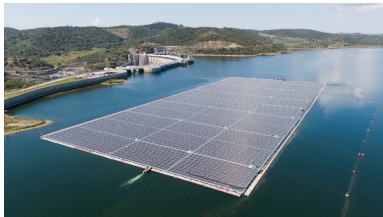
Figure 7.14 Floating PV panels (4 MW) over the Alqueva lake, Alentejo region, Portugal
