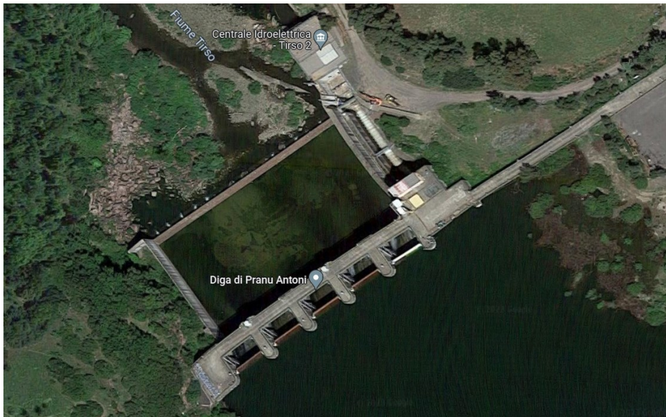
Figure 9.10 Tirso 2 HP plant and Pranu Antoni dam
