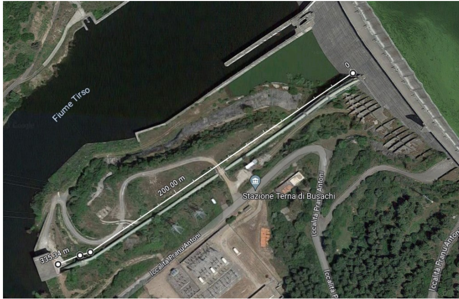
Figure 9.40 Penstock location on the power plant
