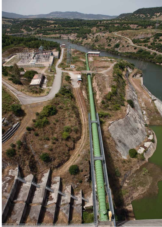
Figure 9.39 Tirso 1 steel penstock
