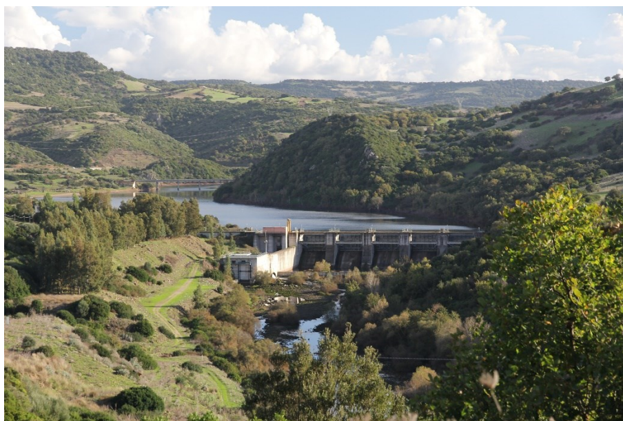
Figure 9.7 Pranu Antoni power dam and power plant
