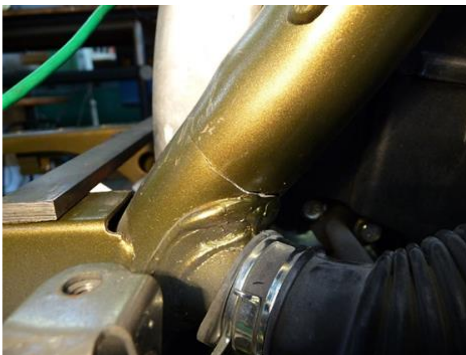
Figure 196 – ActivaD, left weld toe failure at critical point (CPL).
